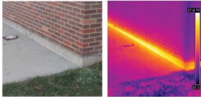
Thermal bridging at slab edge.
